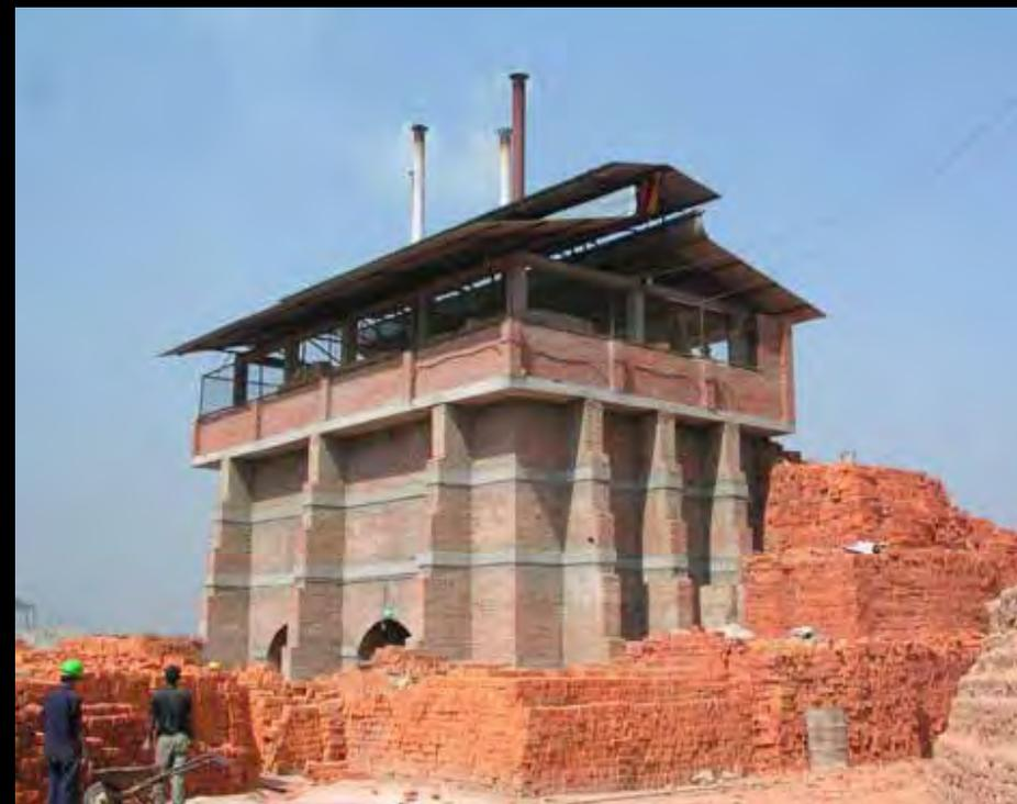
Technologie "VSBK" Vertical Shaft Brick Kiln
